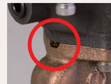
Image. Aperture for leak detection
